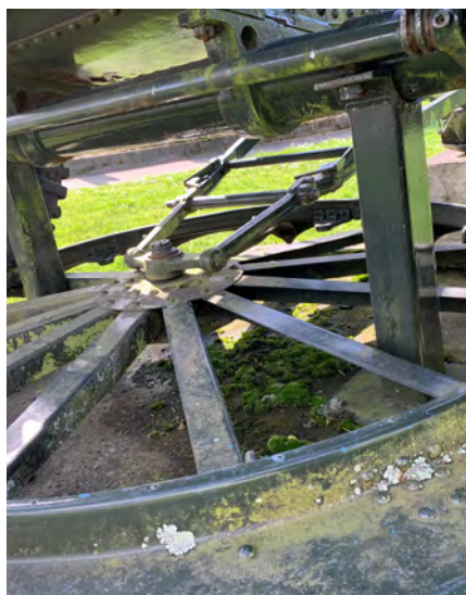
A close-up of the brackets securing the 25-pounder field gun's axle to the concrete plinth.
