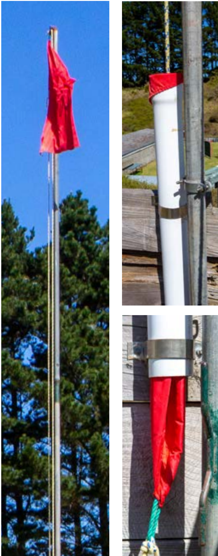
Figure 4.16 Example of red warning flags and containment system
